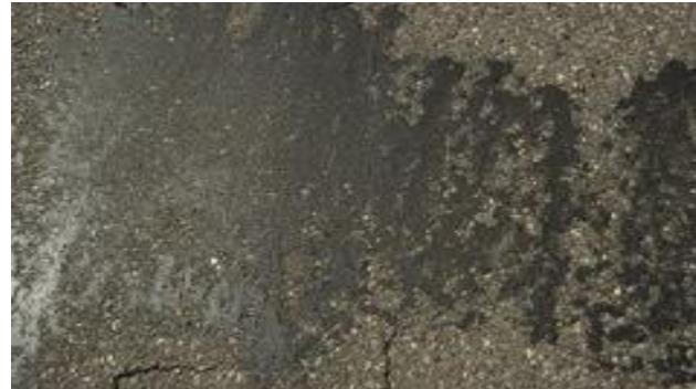
**Edge Cracking** – Running parallel to the road and usually within 1 to 2 feet of the outer edge of the pavement, this distress is caused by traffic loading and weakened base conditions resulting from poor drainage. It is measured in linear feet.
