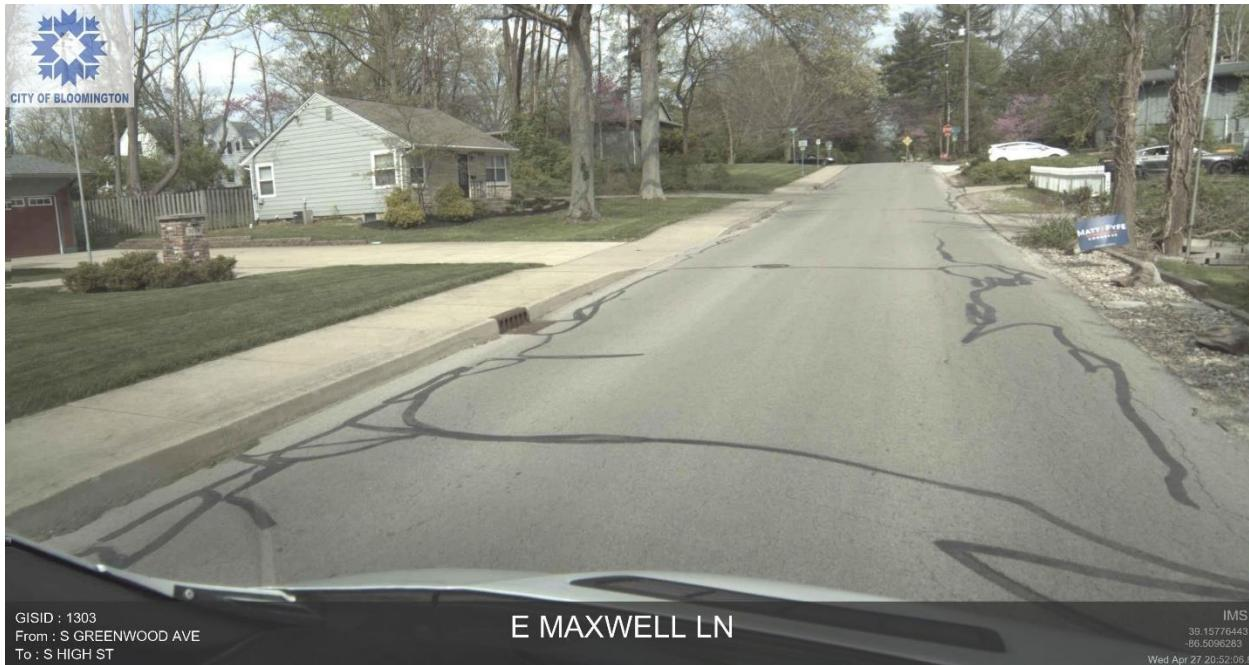
**East Maxwell Lane from South Greenwood Avenue to South High Street (GISID 1303, PCI = 66)** – Rated as Good, the primary cause of deterioration is the longitudinal and transverse cracking, which has been mostly sealed. The pavement surface could be restored further with additional spot patching to fully waterproof the pavement.
