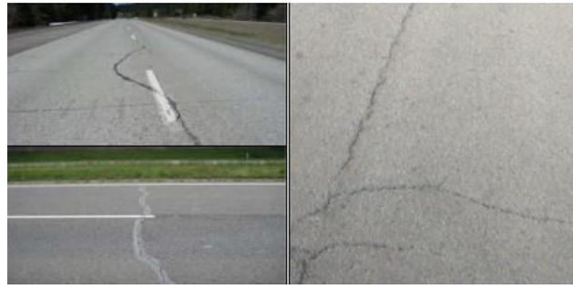
**Block Cracking** – Quantified by their width and square footage, these cracks form interconnected longitudinal and transverse cracks that divide the pavement into approximately rectangular pieces. Block cracking is the result of aging and environmental factors.
