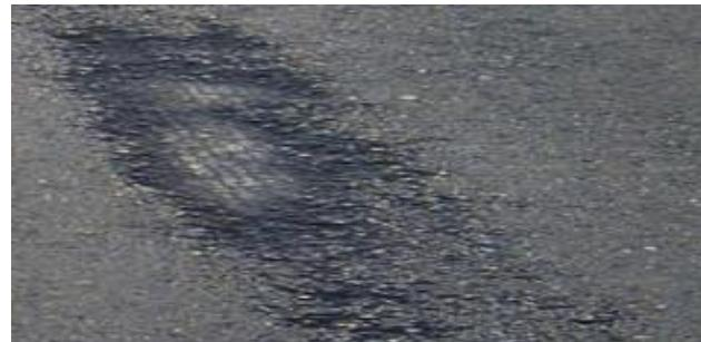
**Bleeding** – This is the presence of free asphalt binder on the roadway surface, which is caused by either an excess of asphalt in the pavement or insufficient voids in the matrix. The result is a pavement surface with reduced skid resistance. This distress is measured by severity and square footage.
