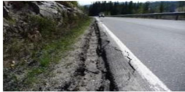
**Distortion** – This includes various localized unevenness in the surface of the pavement including bumps and sags, depressions, swell, corrugation, or shoving. This distress can be caused by a number of factors, including construction issues, subgrade failure, mixture failure, environmental influence, etc.
