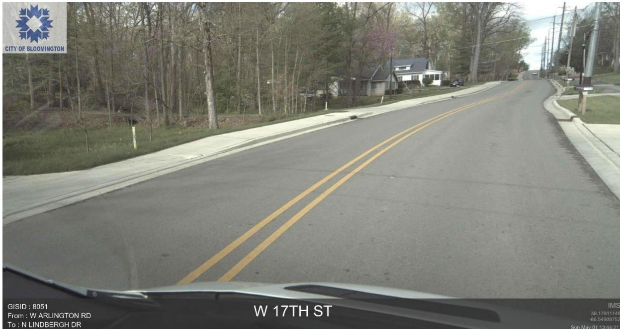
**West 17<sup>th</sup> Street from West Arlington Road to North Lindbergh Drive (GISID 8051, PCI = 78)** – Rated as Very Good, this road displays minor amounts of transverse cracking and raveling. This street is an example of a candidate for preventative maintenance such as microsurfacing to extend the life of the roadway.
