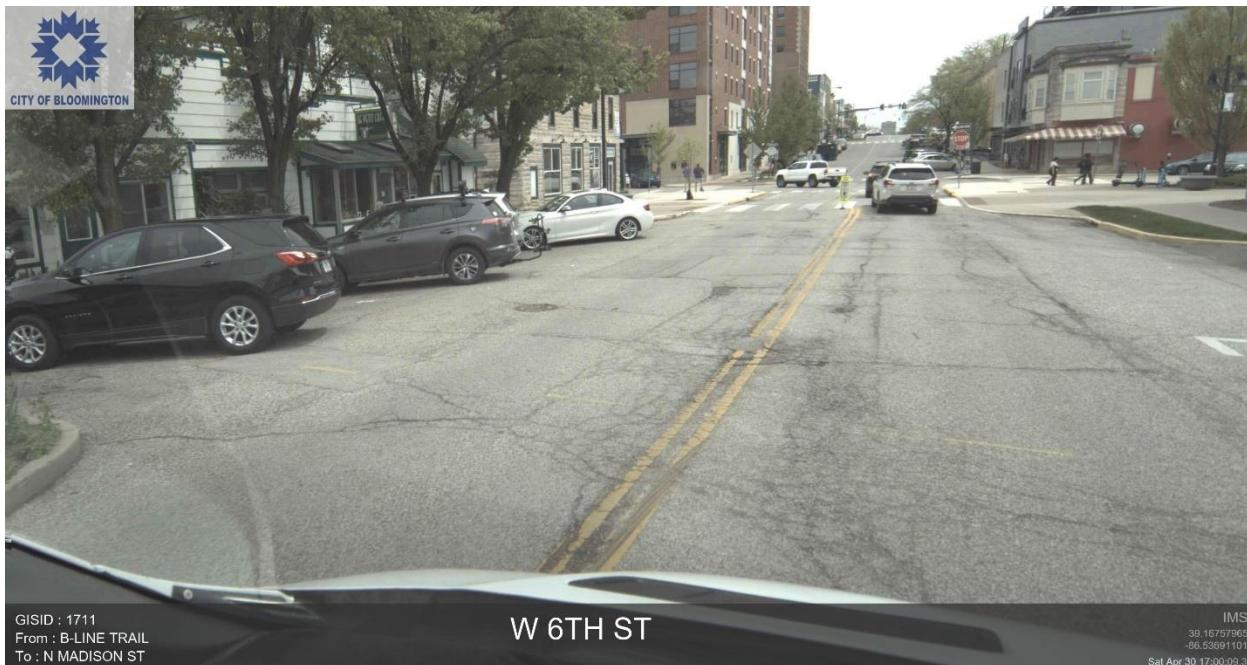
**West 6<sup>th</sup> Street from North Madison Street to B-Line Trail (GISID 1711, PCI = 29)** – Rated as Poor, this segment still has some remaining life before it becomes a critical reconstruction need. As evident in the imagery, a fair amount of the segment displays severe alligator and block cracking. If left untreated, within a short period of time, a partial to full reconstruction would be required.
