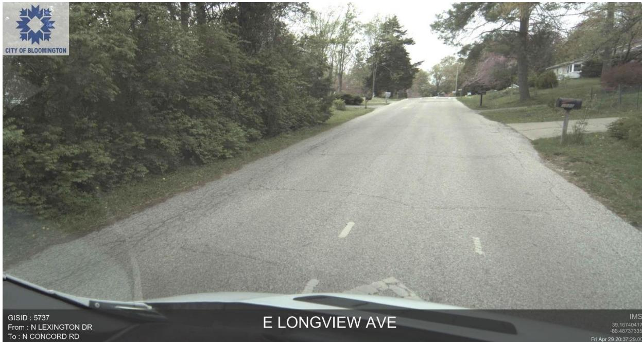
**East Longview Avenue from North Lexington Drive to North Concord Road (GISID 5737, PCI = 44)** – On this street, the primary cause of deterioration is the alligator cracking along the left edge of the pavement. Additionally, transverse cracking is seen throughout the segment.
