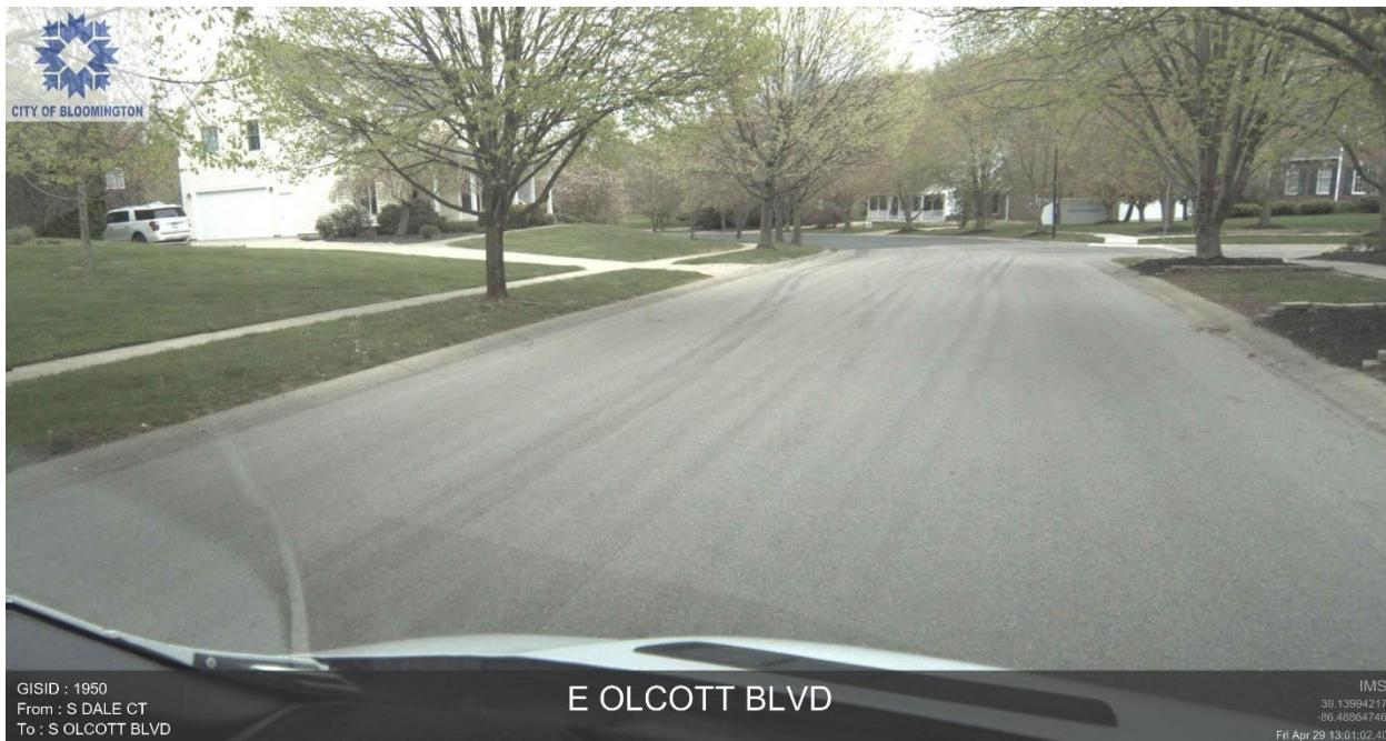
**East Olcott Boulevard from South Dale Court to South Daniel Street (GISID 1950, PCI = 98)** – Rated as Excellent, this pavement displays little to no surface distresses. The ride is smooth, and the surface and the base are intact. Excellent roads should be periodically assessed for crack development that would trigger routine maintenance activities.
