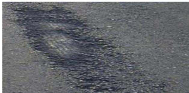
**Bleeding** – This is the presence of free asphalt binder on the roadway surface, which is caused by either an excess of asphalt in the pavement or insufficient voids in the matrix. The result is a pavement surface with reduced skid resistance. This distress is measured by severity and square footage.
