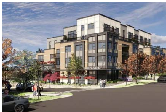
229 S Grant St / The Annex of Bloomington: 102-unit multifamily development with 16 units of workforce housing
