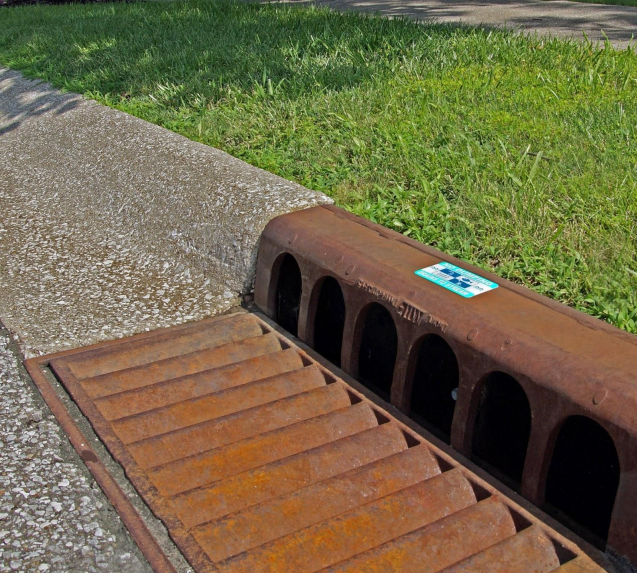
Photo: A storm drain free of debris.
