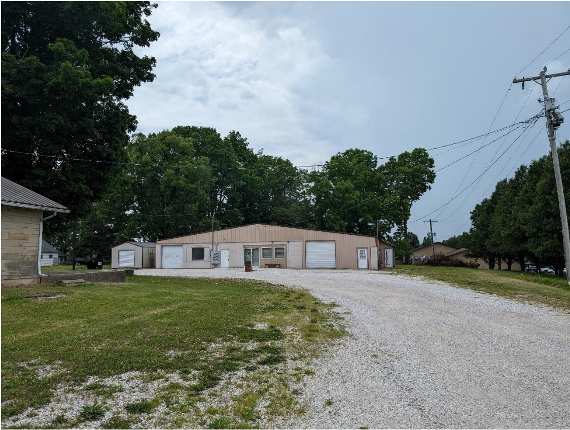
Photo 9: Existing storage building to-be remodeled into Park & Recreational Services – facing west
