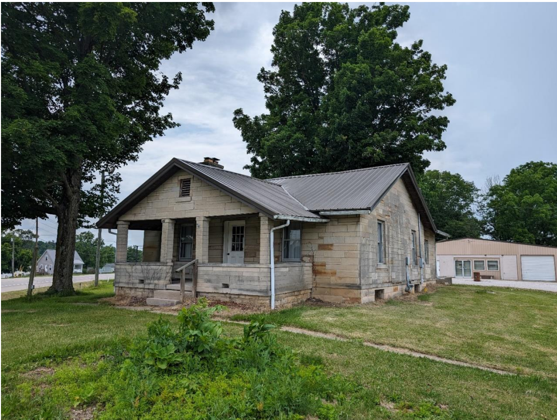
Photo 8: Existing residence to-be remodeled into an office – facing southwest
