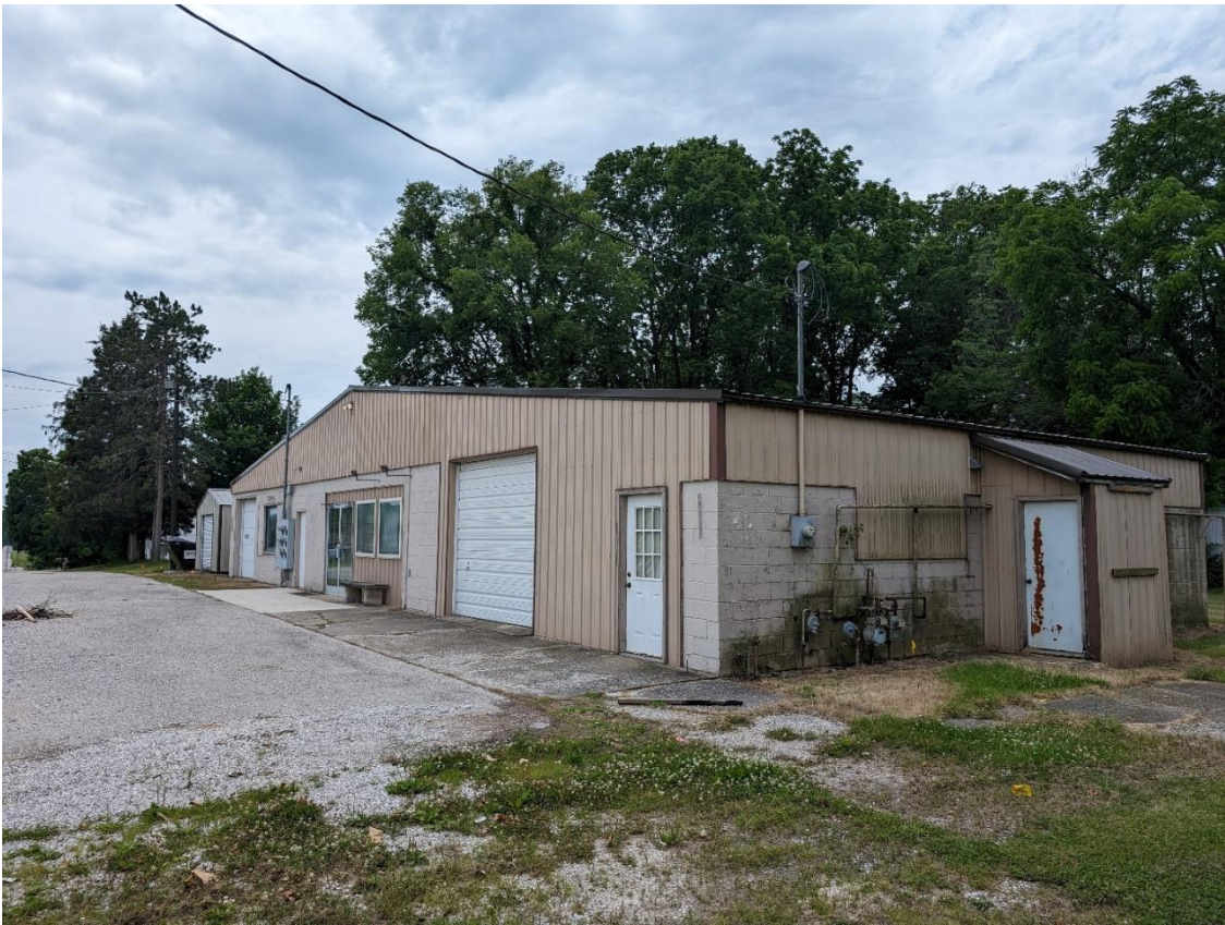
Photo 10: Existing storage building to-be remodeled into an arcade – facing southwest
