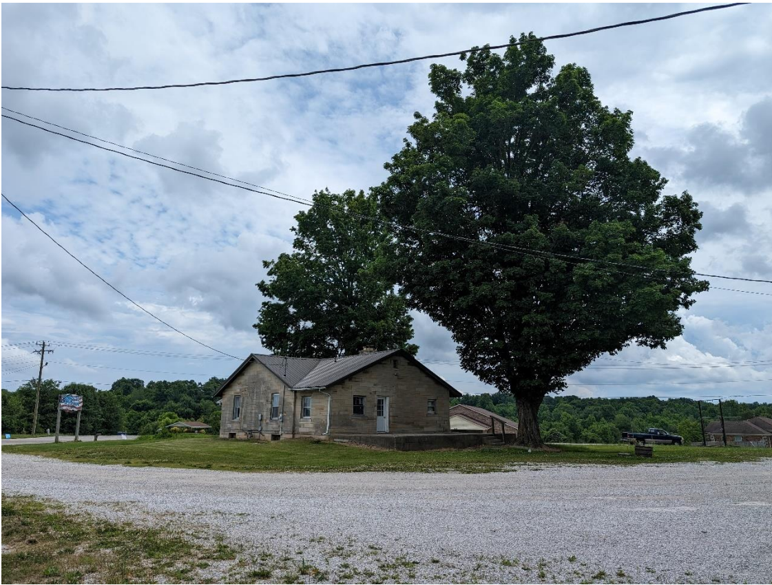
Photo 7: Driveway loop and existing vacant residence to-be remodeled into an office – facing southeast
