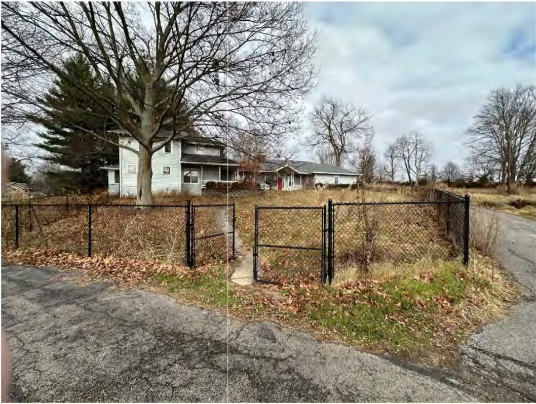
Figure 5. View of single-family residential structure on the property.
