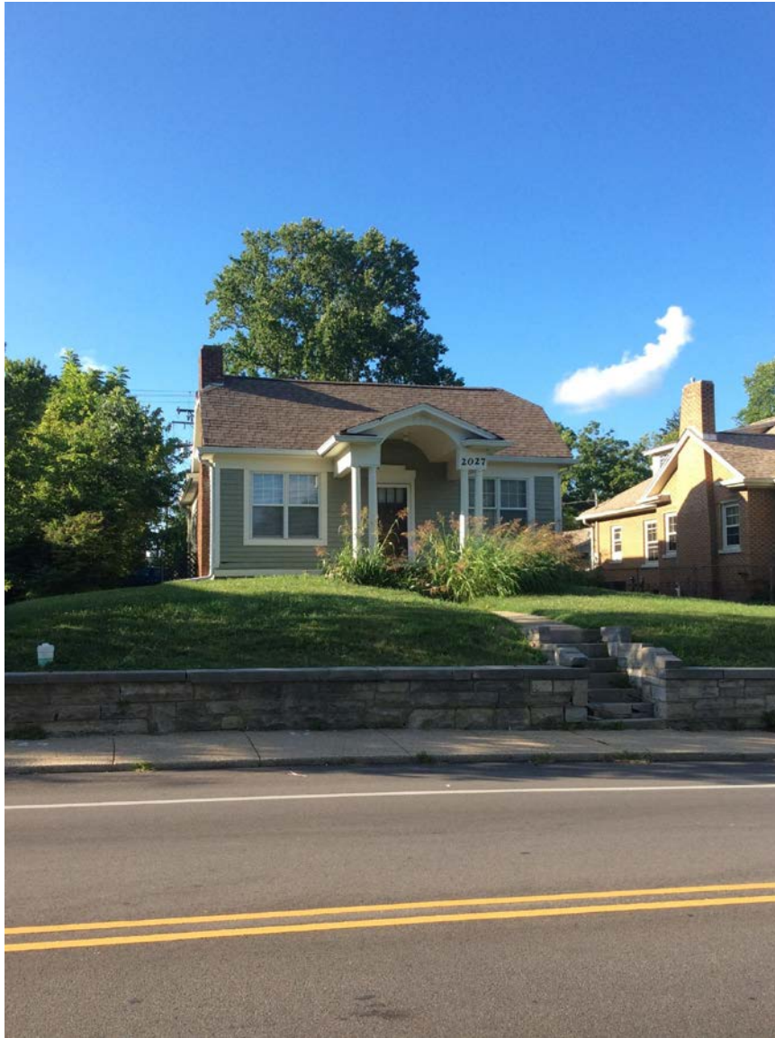
The Rodessa House – 2027 E Third Street - Contributing Architectural Style: Bungalow, 1927
