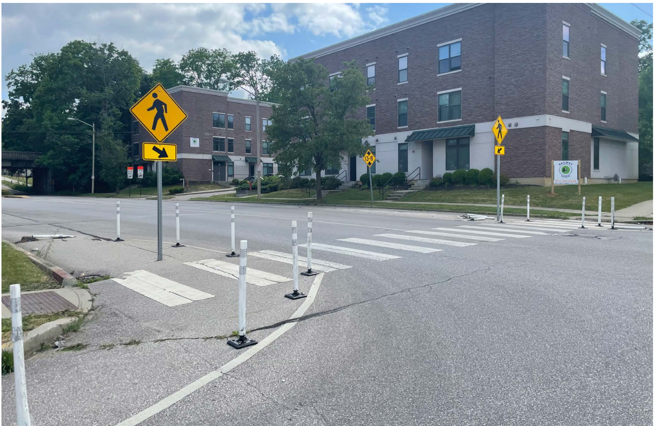
Rapid Implementation Pedestrian Crossing With Curb Extensions Recently Installed at College Ave and 14th St
